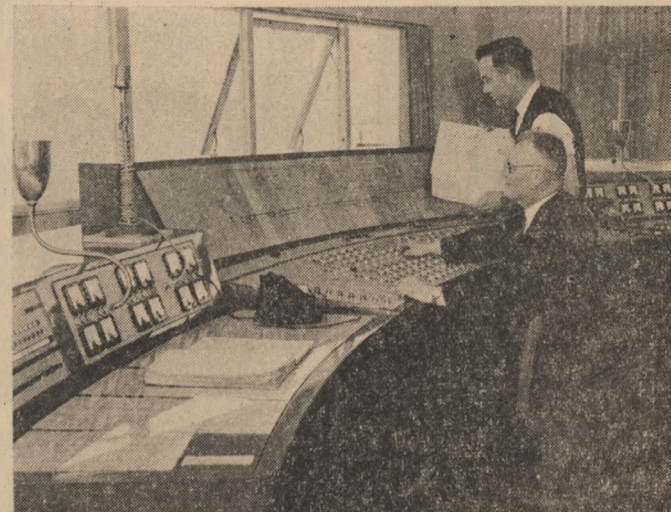
Electrical engineering is a vital force in the modern world of railways. Fingertip control is maintained at Kalwharawhara sub-station of all power supply sub-stations in the Wellington-Paekakariki-Upper Hutt electric traction area. —NZR Publicity photograph
