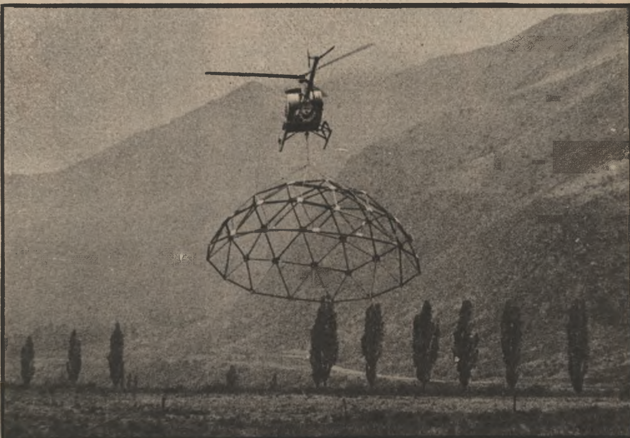
The dome is flown in by helicopter on the first morning
