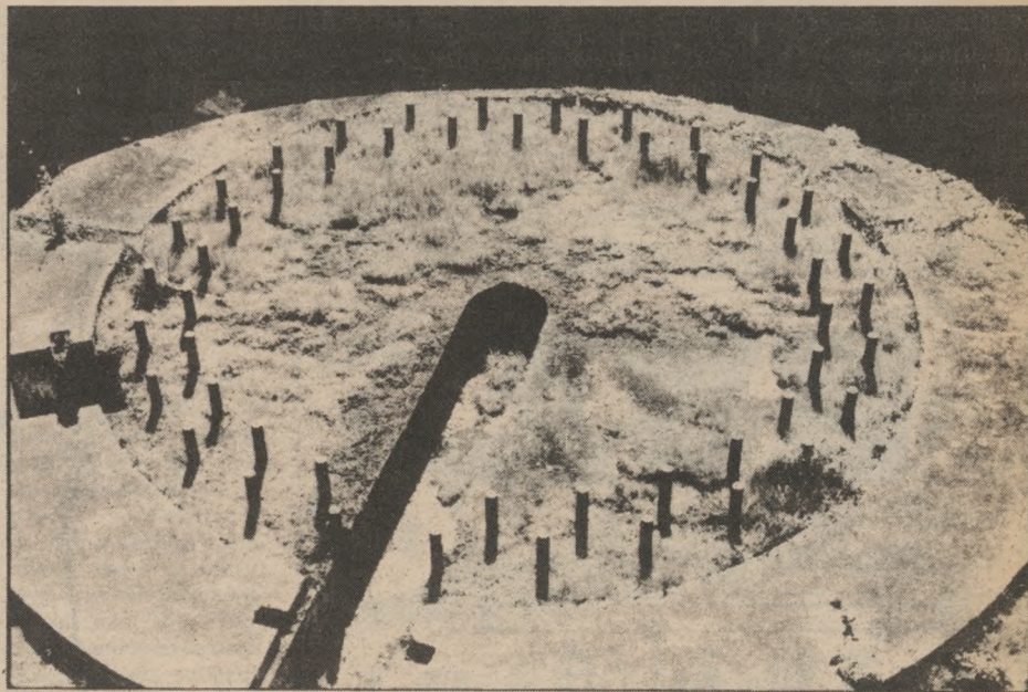
Above : The striking pattern of 52 protruding bolts which formerly anchored the turrets to 2 m thick slab of highly-reinforced concrete. The channel, which extends to the centre of the ring, connects to a machine room and used to contain a drive shaft which transmitted power, enabling the turret to swivel.
